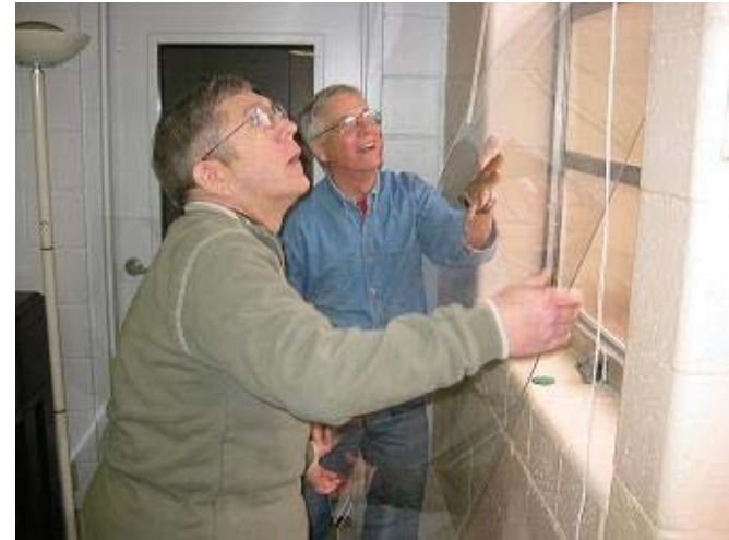
Installing double-paned windows at Bethlehem Lutheran
